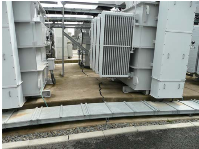
Broken concrete foundation
