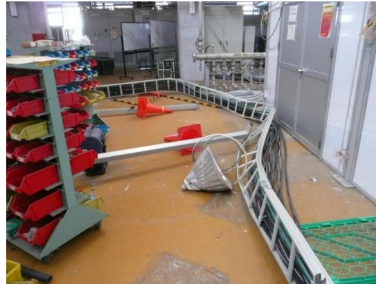
Cable rack falling.
